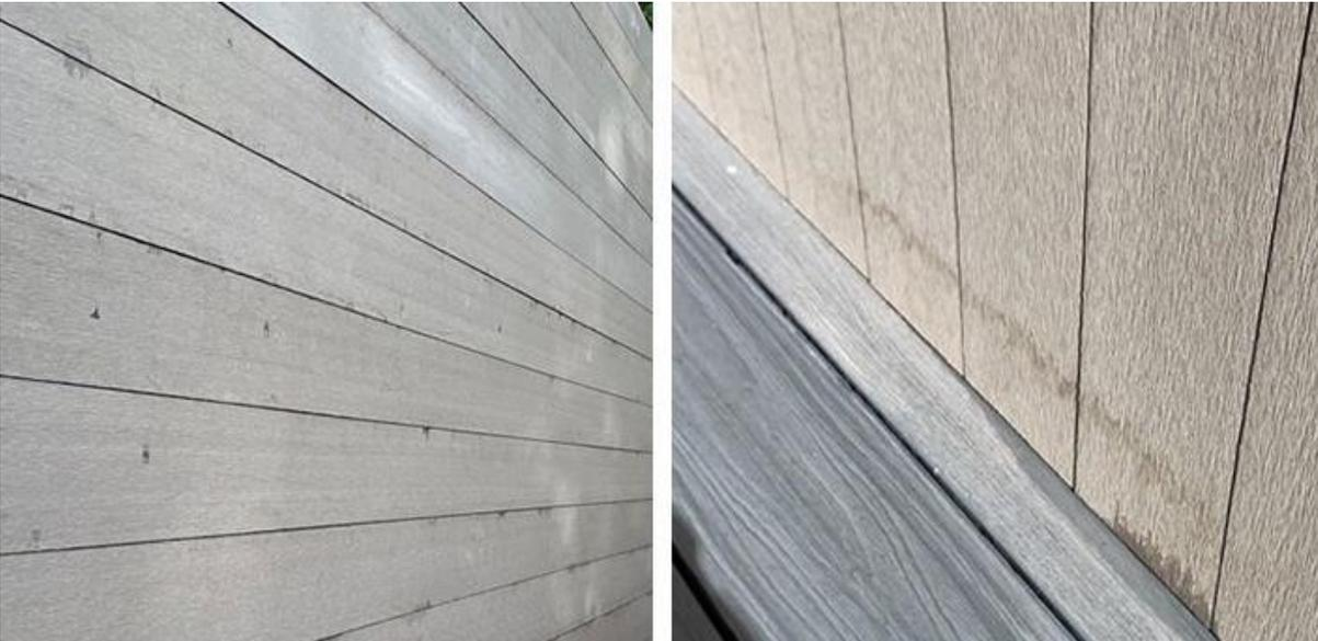
When exposed to UV rays of the sun, they will also continue to undergo some further fading. Extractive bleeding and fading as a result of UV rays is a standard feature of all uncapped composite materials containing wood and will be seen in products across the market.
