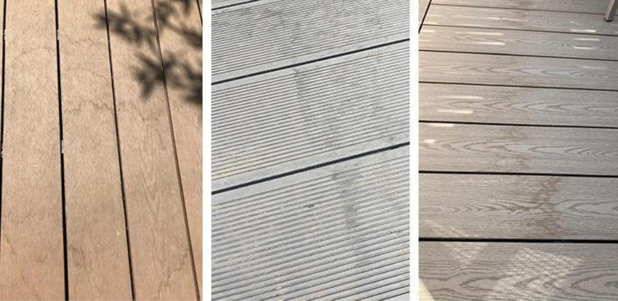
After the natural process of extractive bleeding, the boards are subject to standard weathering, primarily from the UV rays of the sun. Our boards contain a UV stabiliser, but will undergo some further fading. The most noticeable change is when using the wood grain effect where the contrast between the two shades decreases significantly.
